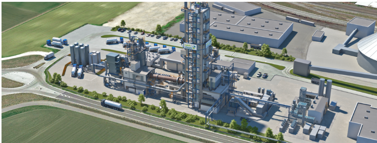
Figure 21 : Illustration of the oxyfuel plant for the "catch4climate" demonstration project in Mergelstetten.
