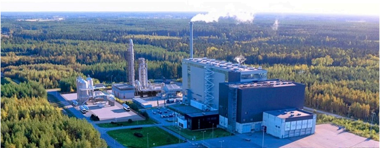
Westenergy waste incineration plant in Finland with CO 2 capture system
